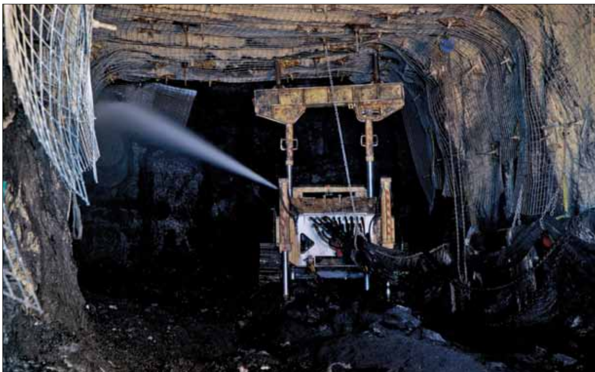
Figure 12.2: Hydro monitor at work 3
