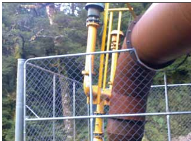
Figure 9.4: Gas riser and slimline shaft 45
