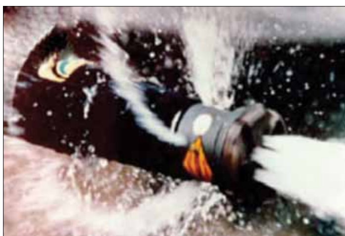
Figure 9.3: Rotating drill bit with high-pressure water 34
