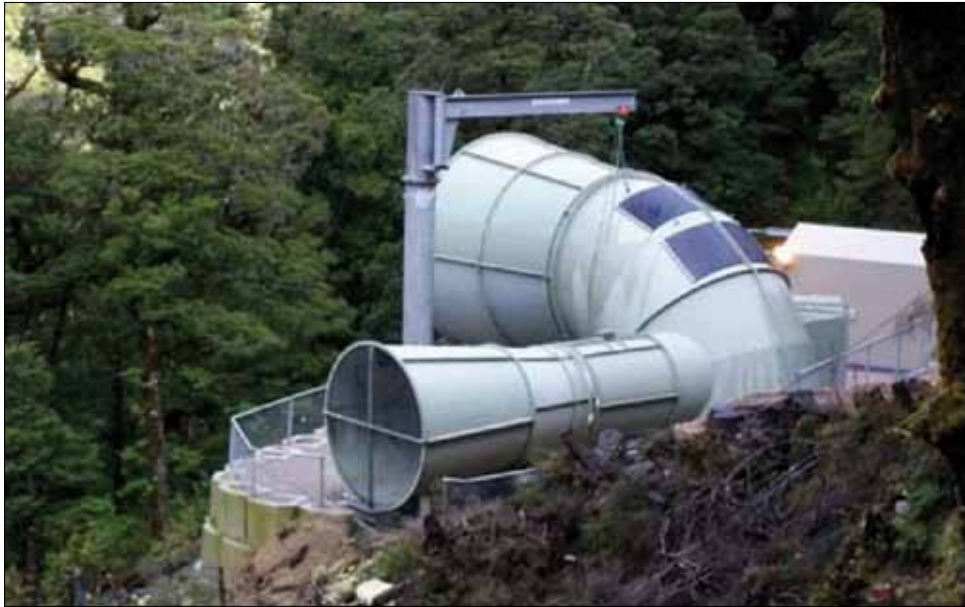
Figure 8.5: The surface back-up fan
