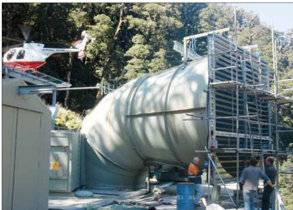
Figure 8.7: Easé showing louvres being installed
